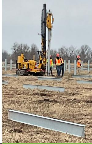
▲ Support posts for solar panels are driven into the ground at what will become the 200 MW Huck Finn Renewable Energy Center. Construction is expected to be complete at the end of 2024. Ameren Missouri is set to acquire the facility upon completion. It will become the company's largest solar facility to date, anticipated to supply the energy needs of more than 37,000 Ameren Missouri residential customers.
