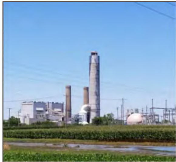
Sioux Energy Center
