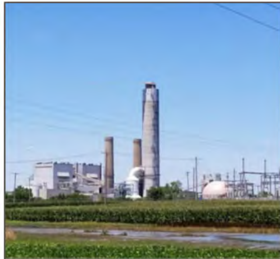
Sioux Energy Center
