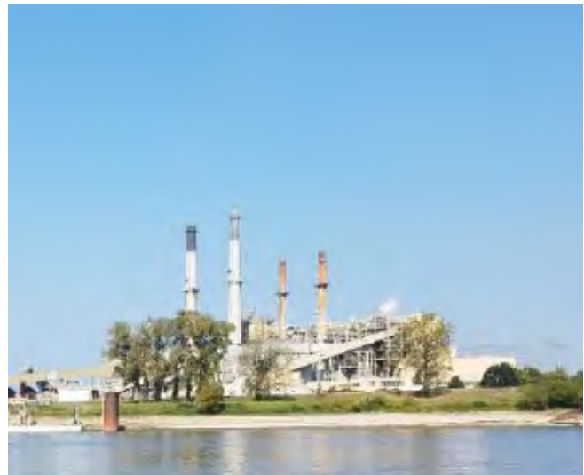
Meramec Energy Center
