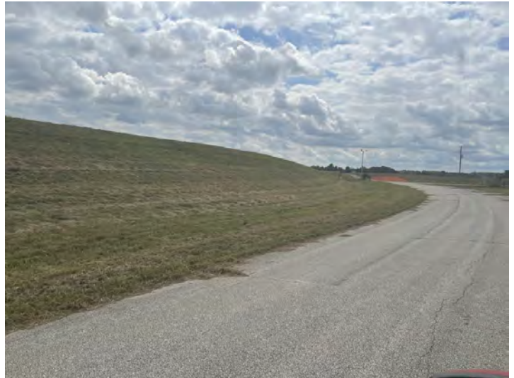
West embankment (facing S)
