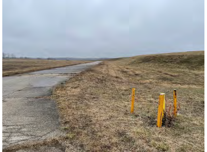
East embankment (facing S)
