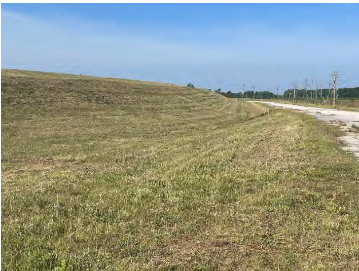
North embankment (facing SW)
