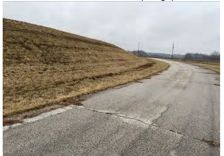
West embankment (facing S)
