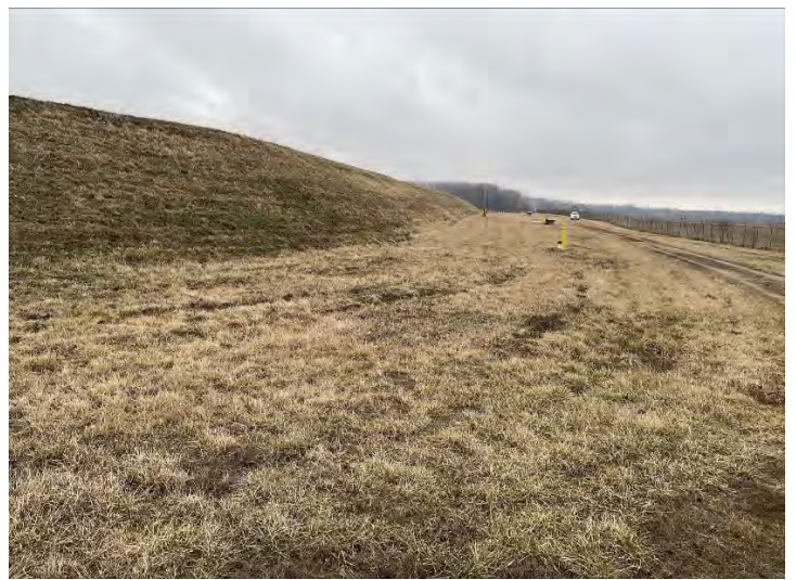
South embankment (facing E)
