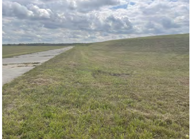
East embankment (facing S)
