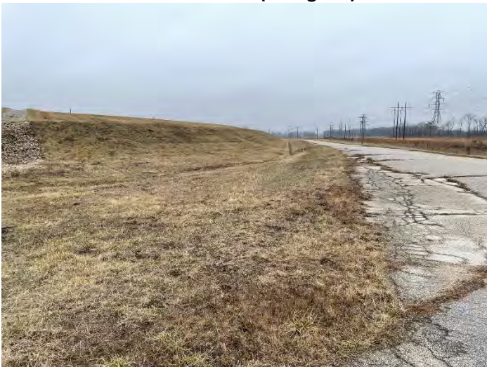
North embankment (facing SW)
