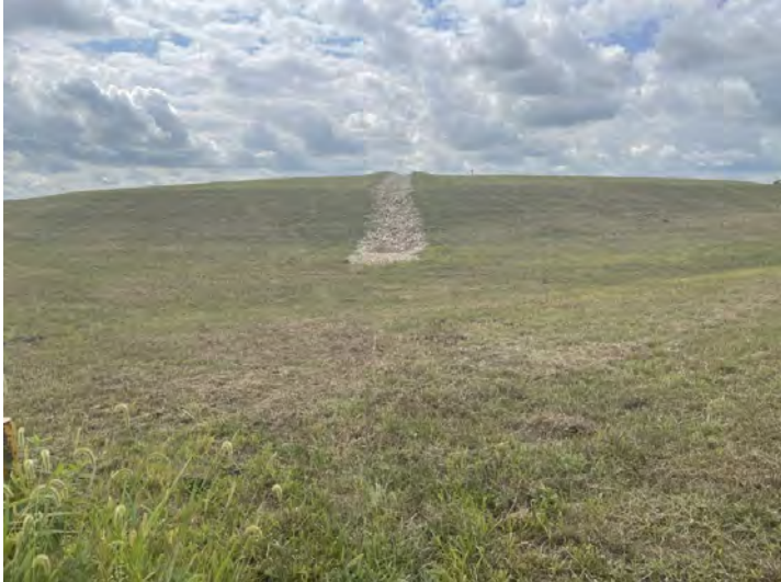
North letdown (facing SW)
