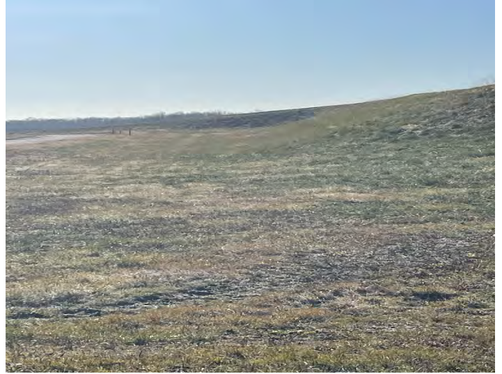
East embankment (facing S)
