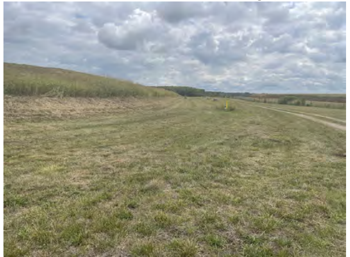
South embankment (facing E)
