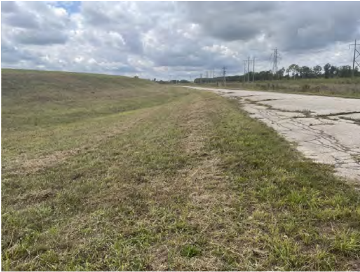
North embankment (facing SW)
