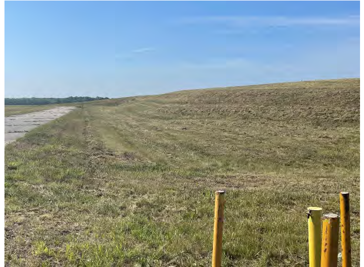
East embankment (facing S)
