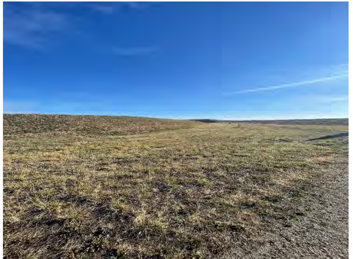
South embankment (facing E)
