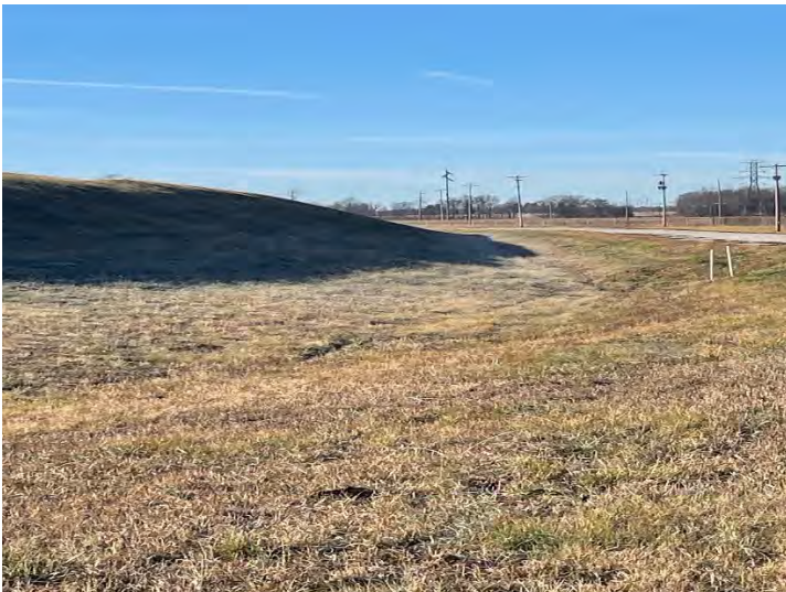
North embankment (facing SW)
