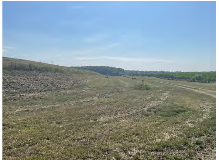
South embankment (facing E)
