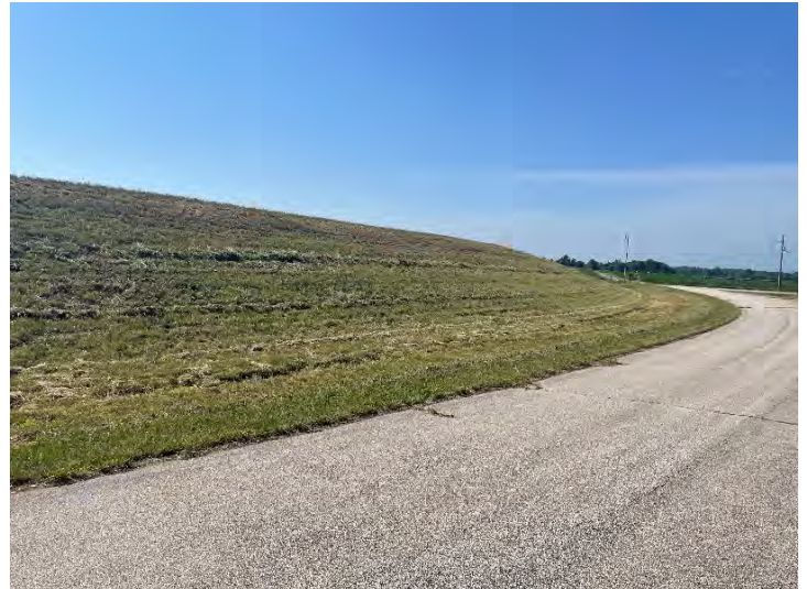
West embankment (facing S)
