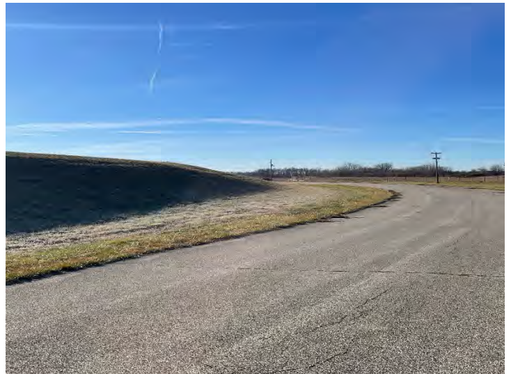
West embankment (facing S)
