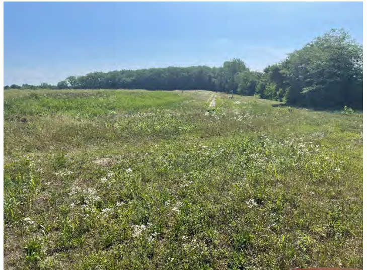
South embankment and outfall trench (facing E)
