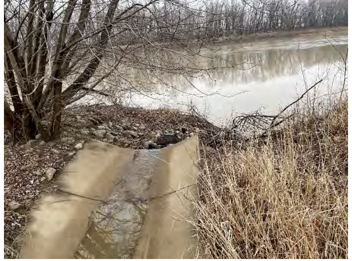
Outfall Discharge (facing east)
