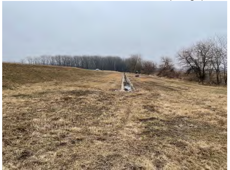
South embankment and outfall trench (facing E)
