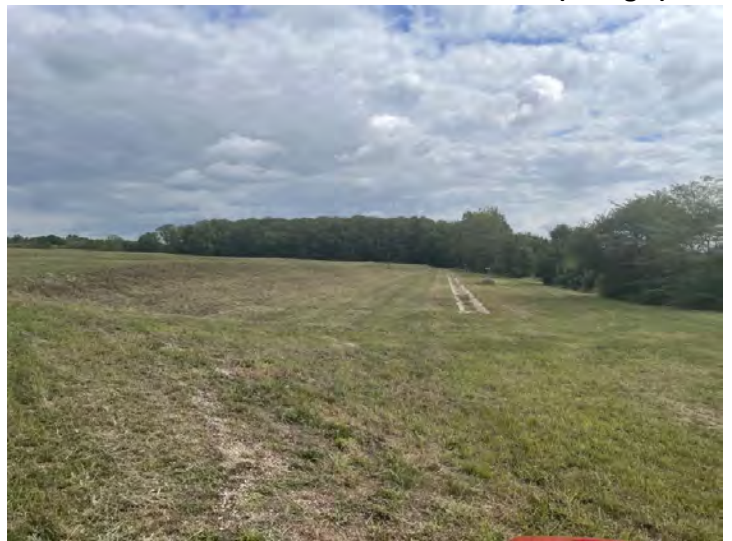
South embankment and outfall trench (facing E)
