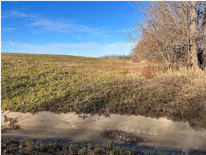
East (river) embankment (facing N)
