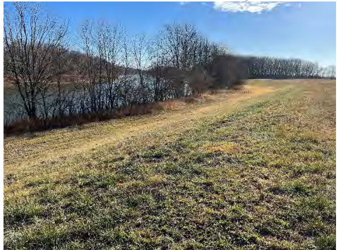
East (river) embankment (facing S)
