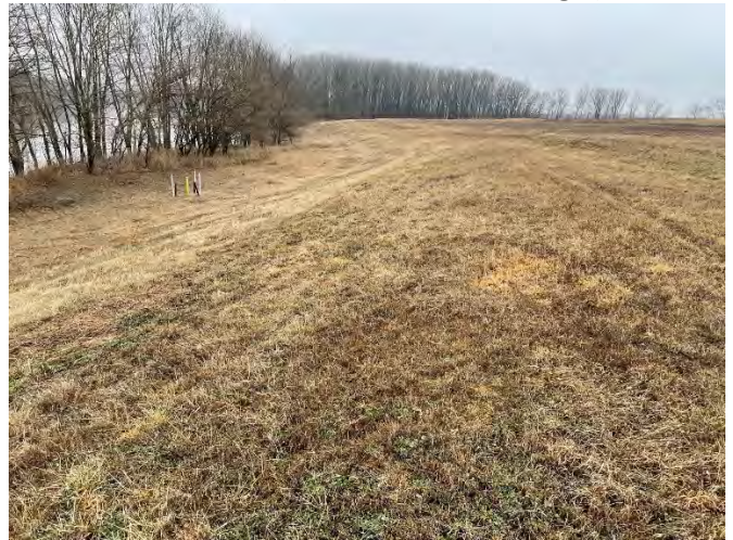
East (river) embankment (facing S)
