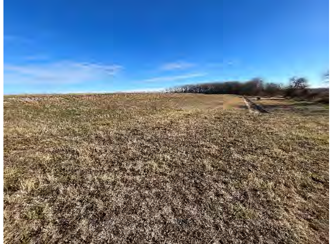
South embankment and outfall trench (facing E)
