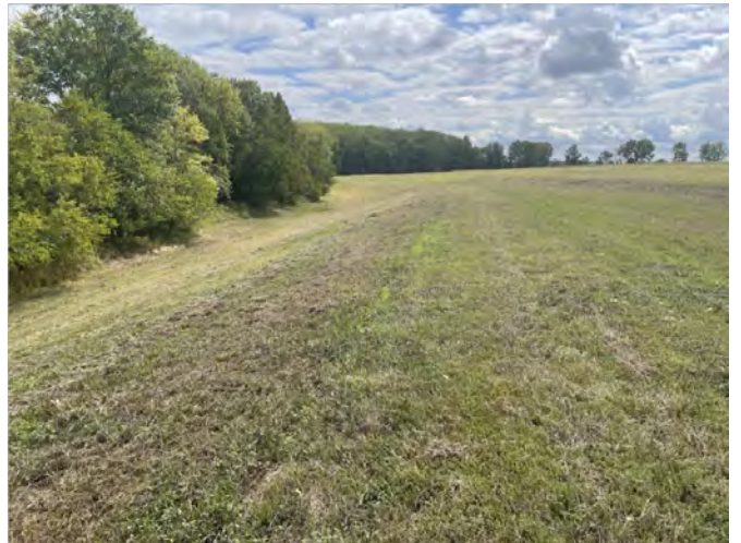
East (river) embankment (facing S)
