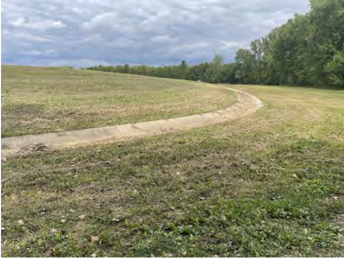
Outfall drainage trench (facing N)
