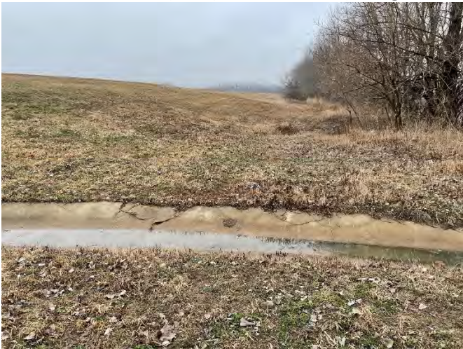
East (river) embankment (facing N)
