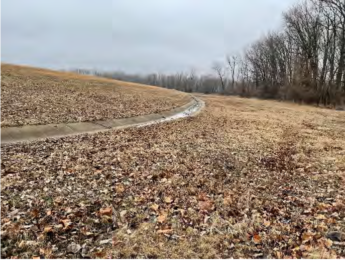
Outfall drainage trench (facing N)
