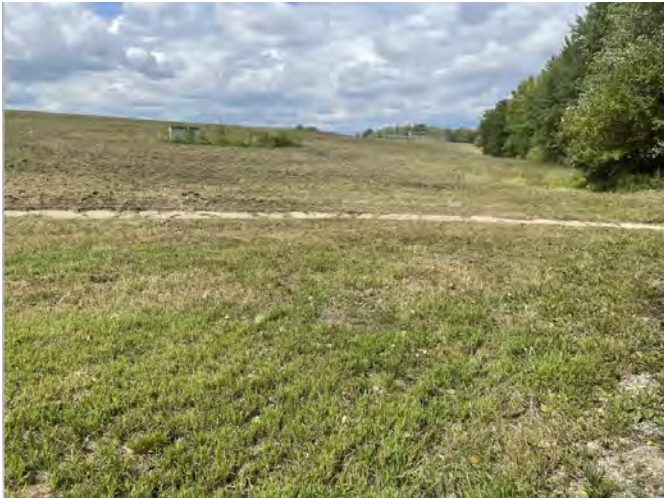
East (river) embankment (facing N)
