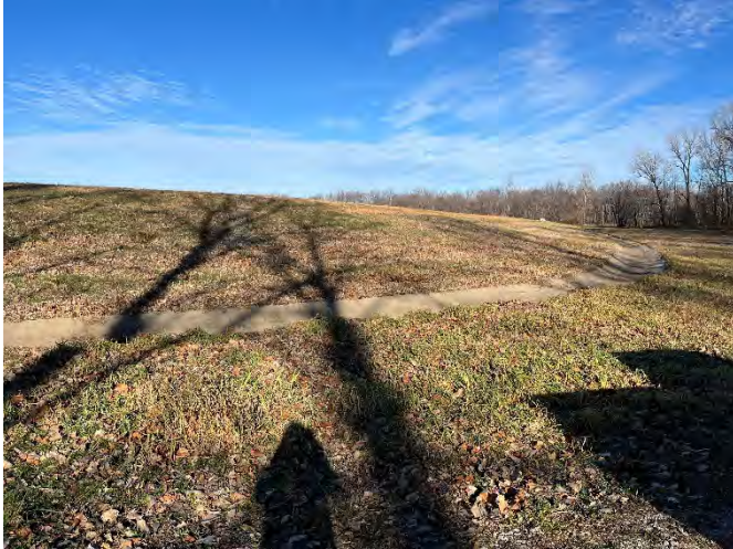
Outfall drainage trench (facing N)
