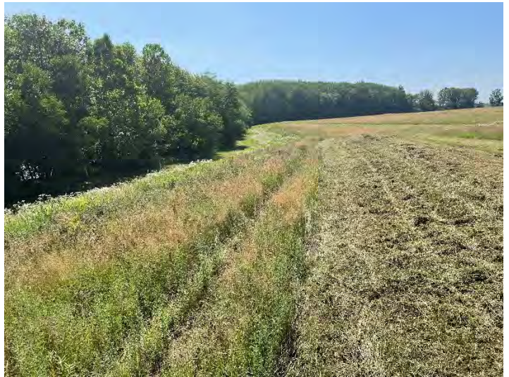
East (river) embankment (facing S)
