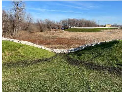
Fly Ash Pond Cap – Outlet 5 and embankment (looking east and west)
