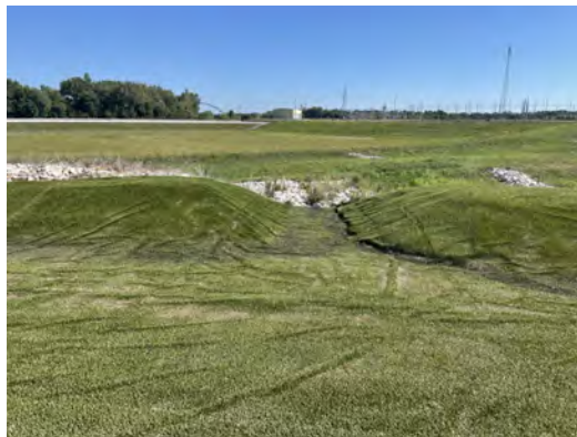
Fly Ash Pond Cap – Outlet 6 and embankment (facing east and west)
