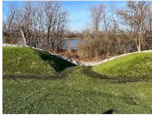
Fly Ash Pond Cap – Outlet 3 and embankment (facing north and south)
