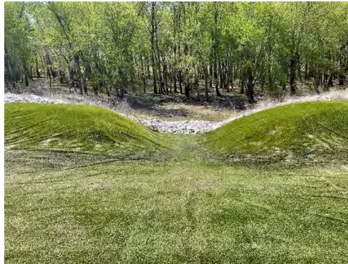
Fly Ash Pond Cap – Outlet 1 and embankment (facing east and west)
