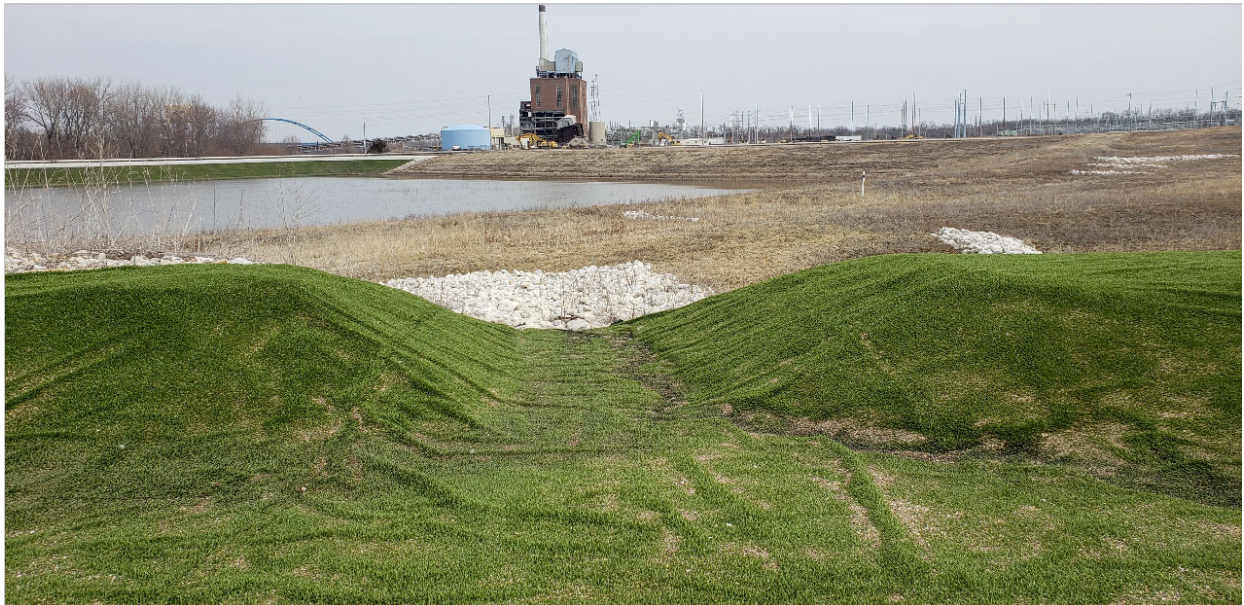
Fly Ash Pond Cap – outlet 6
