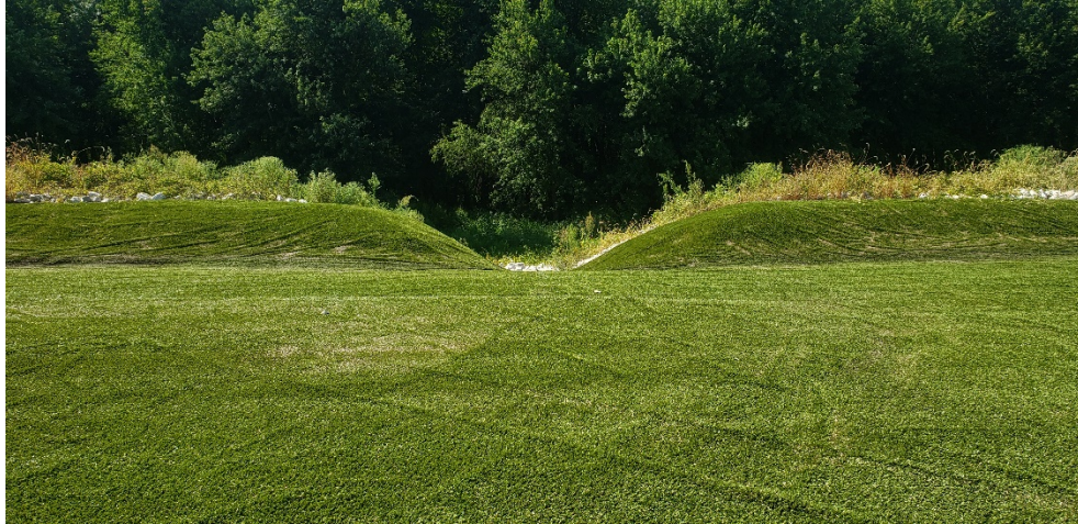
Fly Ash Pond Cap – Outlet 1 and embankment (facing east and west)
