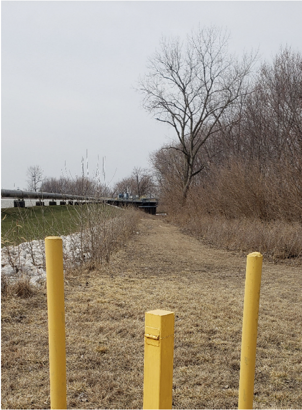
Bottom Ash embankment north side by well 9
