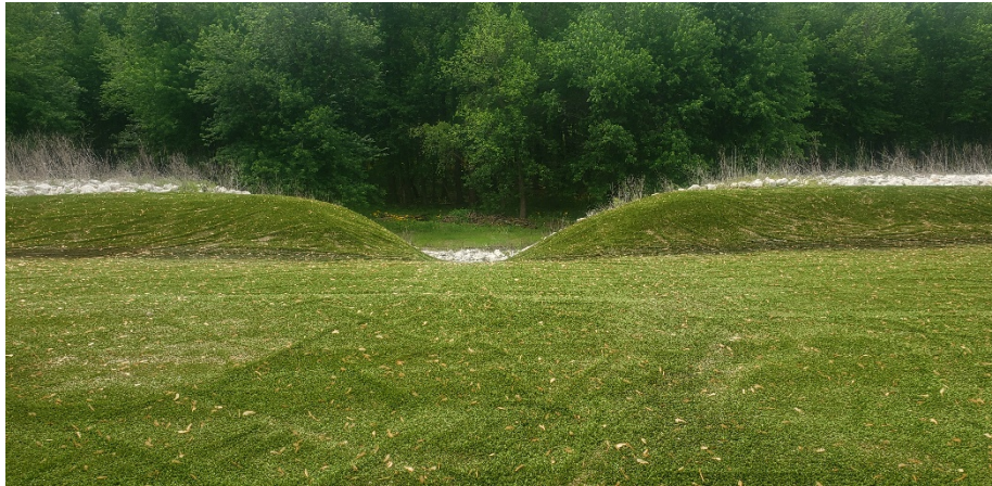
Fly Ash Pond Cap – Outlet 1 and embankment (facing west and north)
