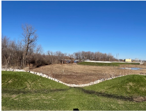
Fly Ash Pond Cap – Outlet 5 and embankment (looking east and west)
