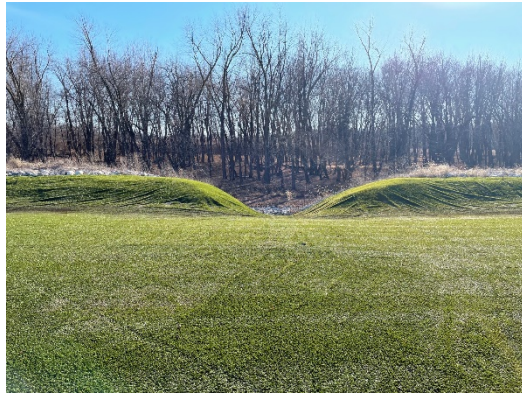
Fly Ash Pond Cap – Outlet 1 and embankment (facing east and west)
