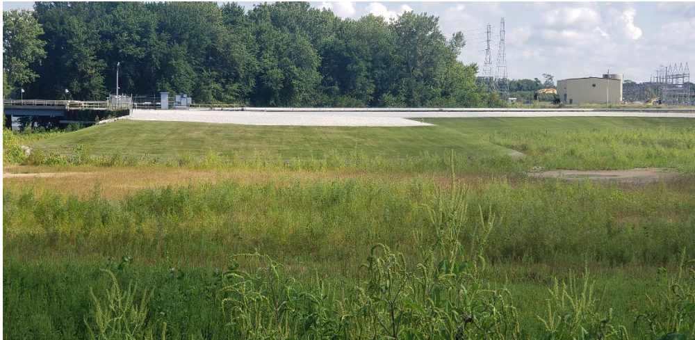
Bottom Ash CAP - embankment view (facing north)
