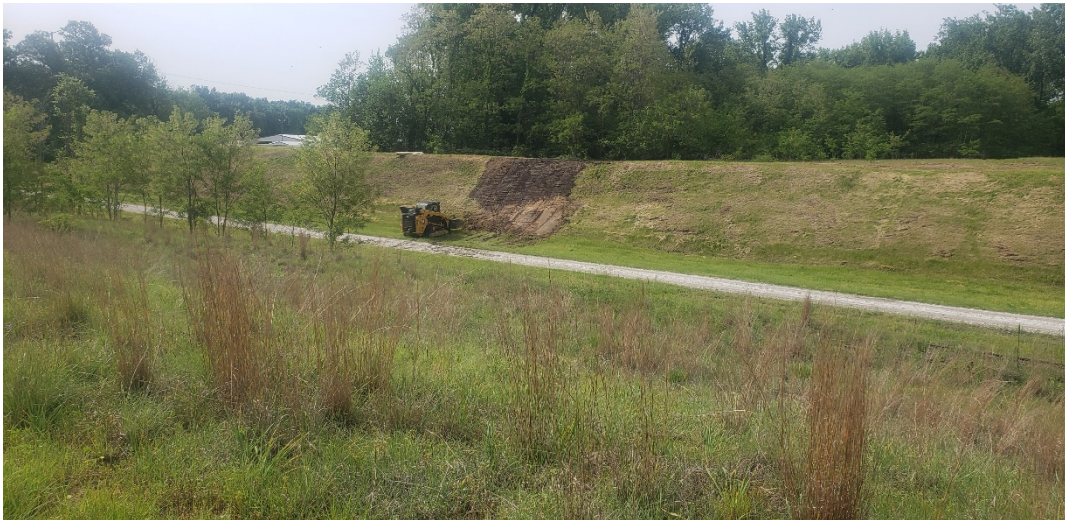
REPAIRED MAY 2022 - Old East Pond north side embankment washout
