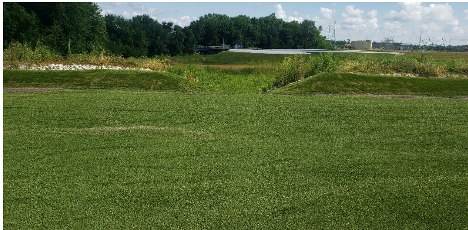
Fly Ash Pond Cap – Outlet 5 and embankment (looking east and west)
