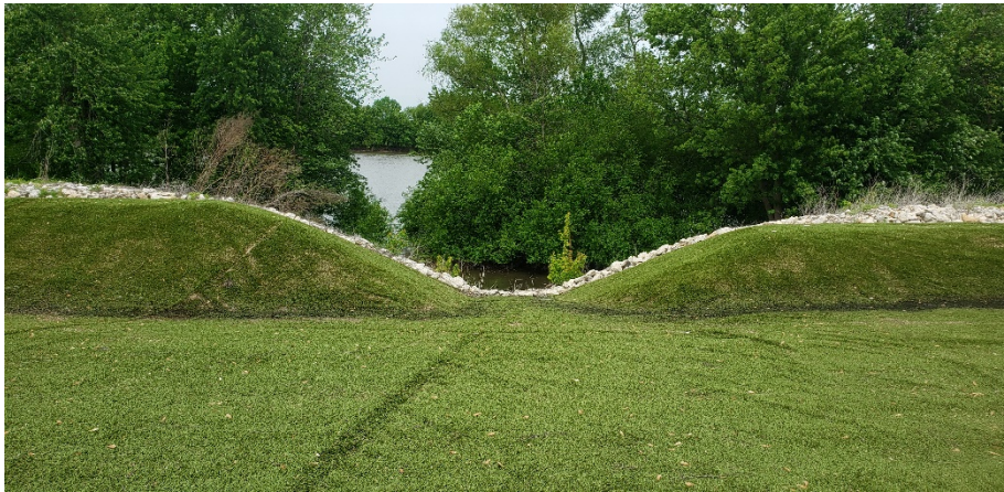
Fly Ash Pond Cap – outlet 3 and embankment (facing north and south)
