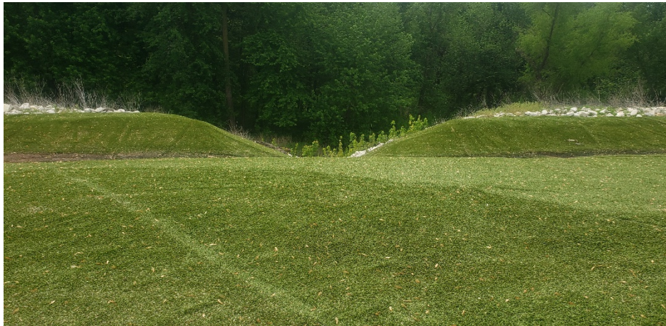
Fly Ash Pond Cap – outlet 2 and embankment (facing east and west)
