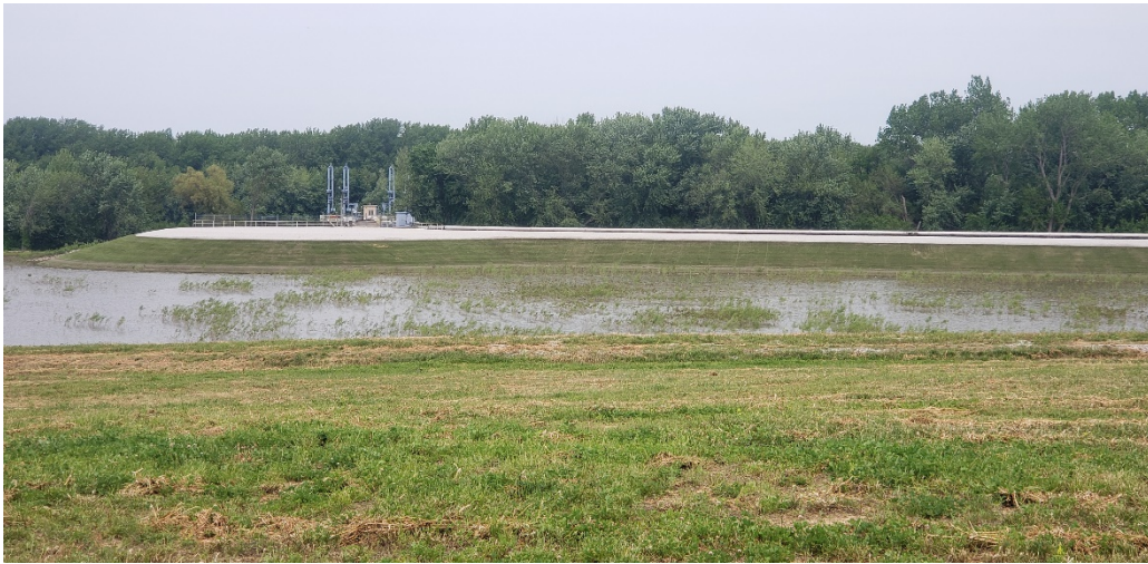
Bottom Ash CAP - embankment view (facing north)
