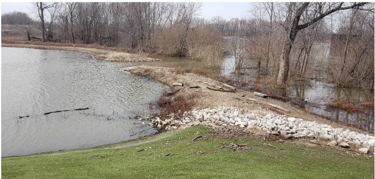
Bottom Ash embankment outlet to river
