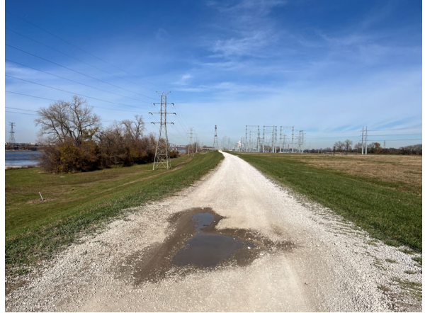
West Embankment, center section
