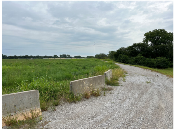
South Embankment, facing east
