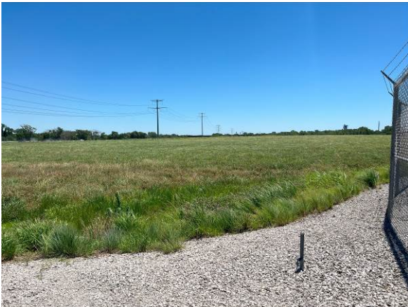
North Pump Station, facing south
