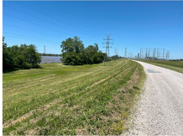
West Embankment, center section
