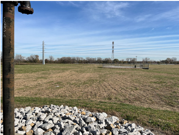
North Pump station, facing east
