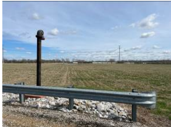
South Pump station, facing east
