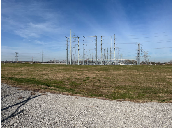
North Pump Station, facing north
