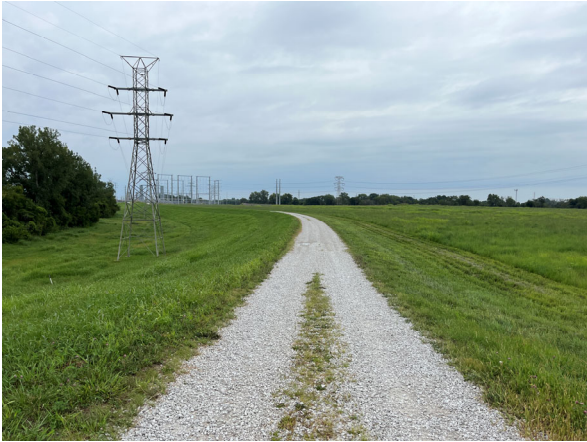
West Embankment, south section
