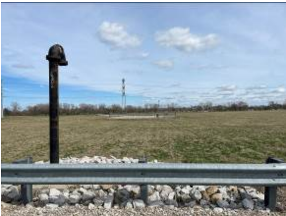
North Pump station, facing east
