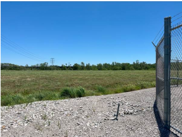
South Pump Station, facing south
