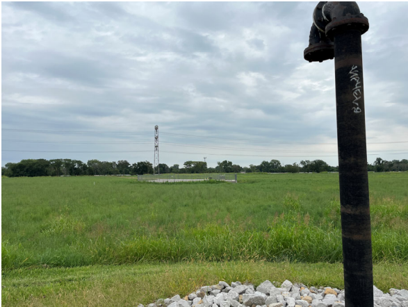
North Pump station, facing east
