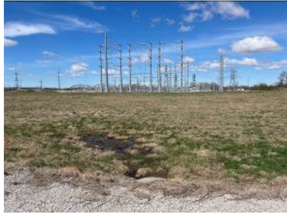
North Pump Station, facing north
