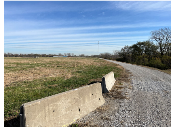
South Embankment, facing east
