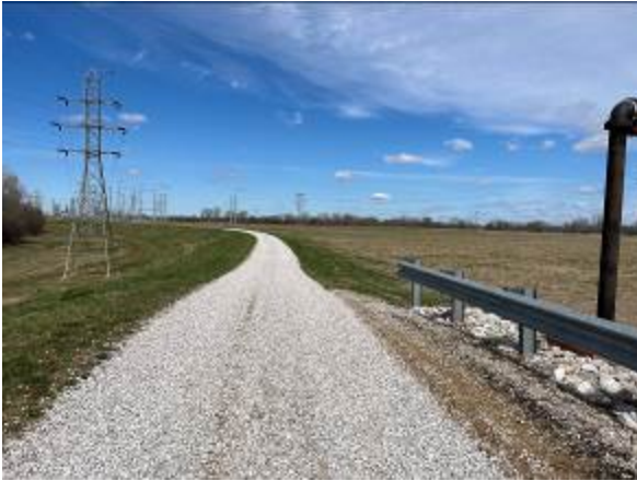
West Embankment, south section
