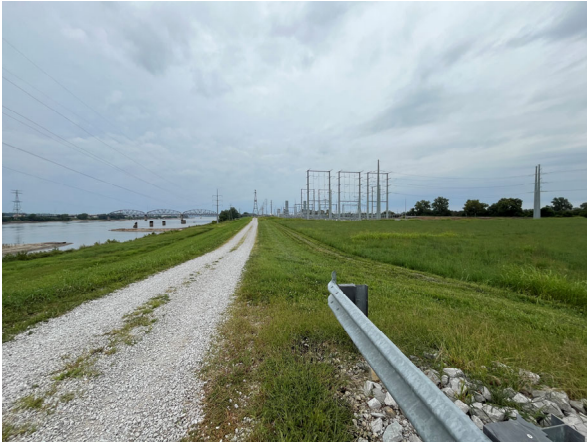
West Embankment, north section
