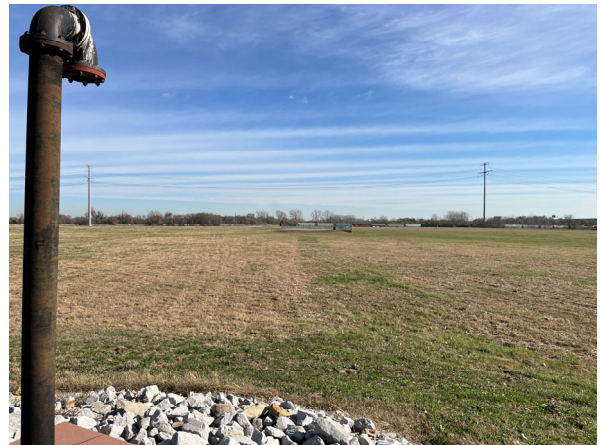
South Pump station, facing east
