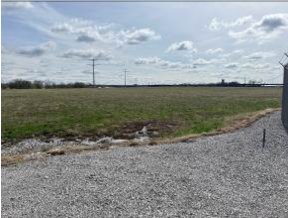
North Pump Station, facing south
