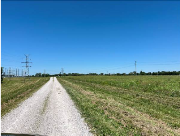
West Embankment, south section
