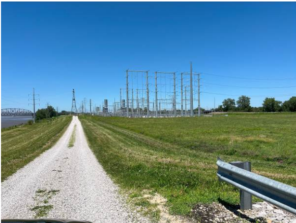
West Embankment, north section
