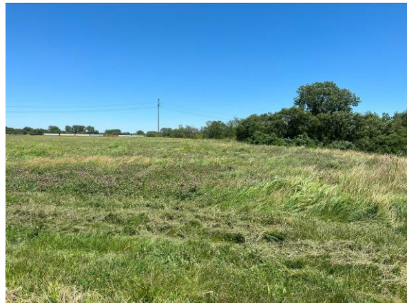
South Embankment, facing east
