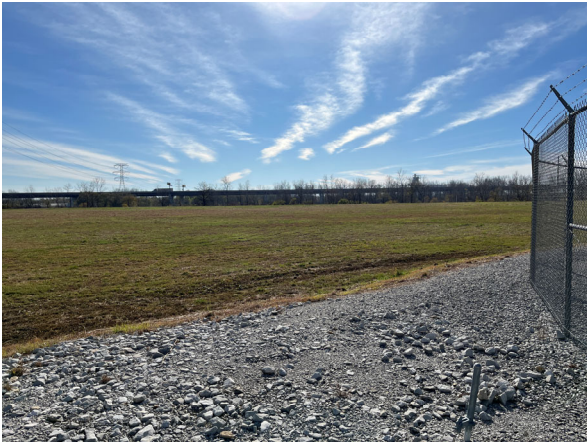
South Pump Station, facing south
