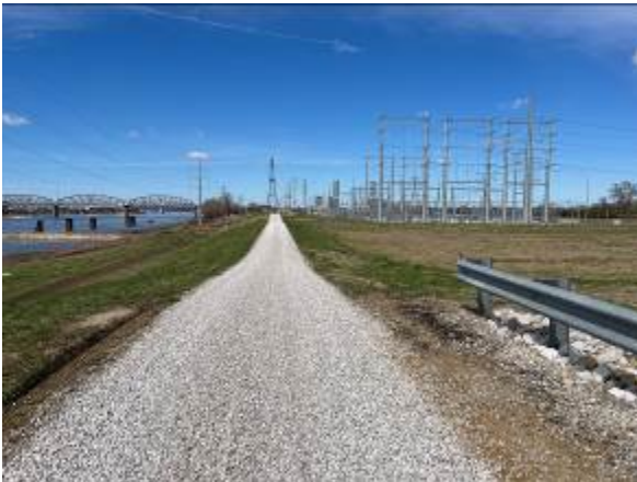
West Embankment, north section
