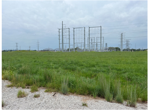
North Pump Station, facing north
