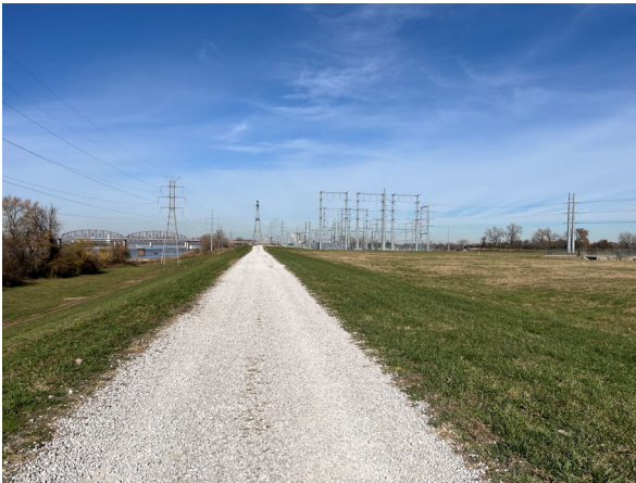
West Embankment, north section
