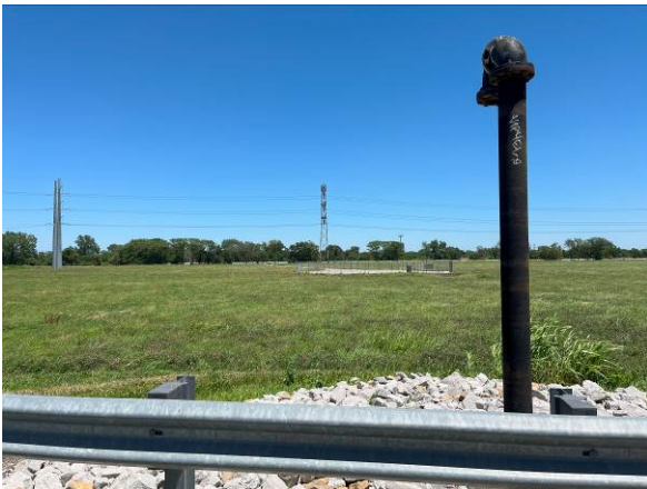
North Pump station, facing east
