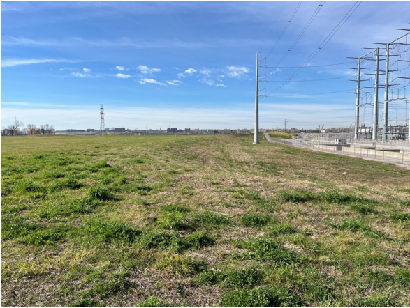
North embankment, facing west
