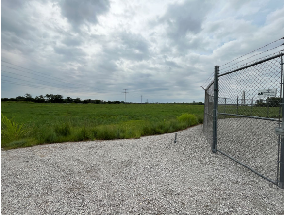
North Pump Station, facing south
