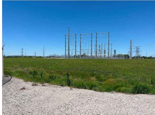
North Pump Station, facing north
