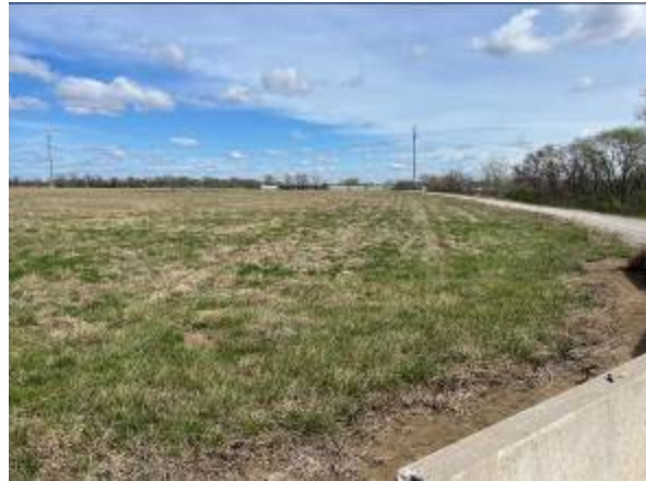
South Embankment, facing east
