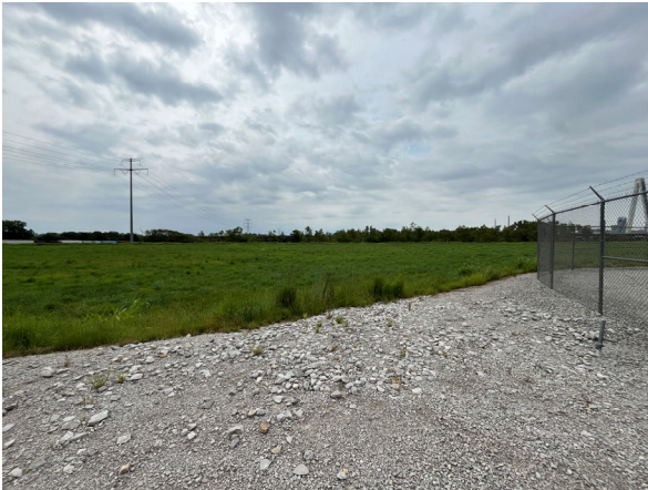
South Pump Station, facing south
