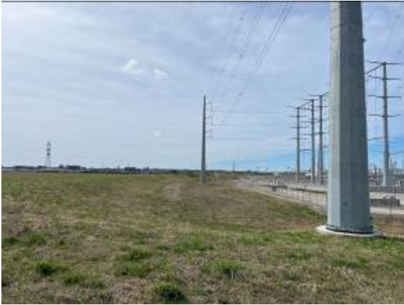
North embankment, facing west
