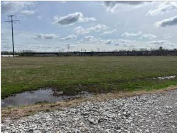
South Pump Station, facing south
