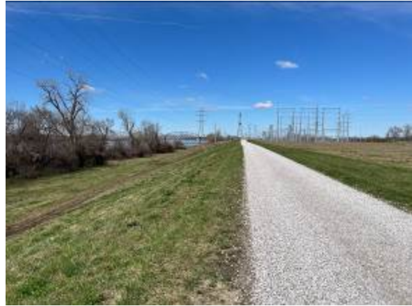
West Embankment, center section
