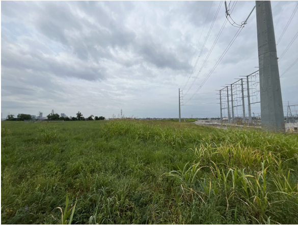
North embankment, facing west
