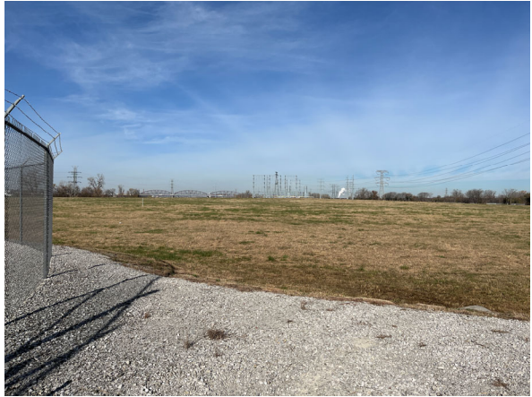
South Pump Station, facing north
