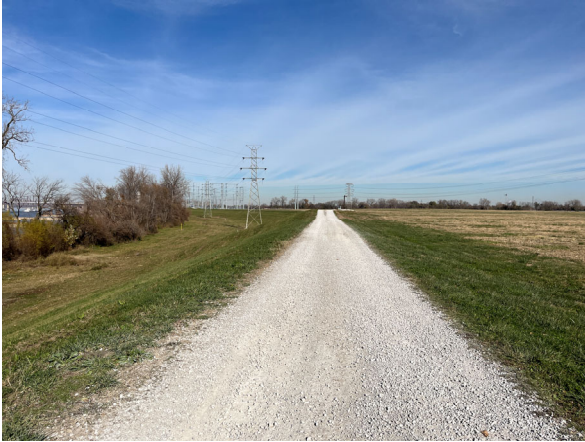
West Embankment, south section
