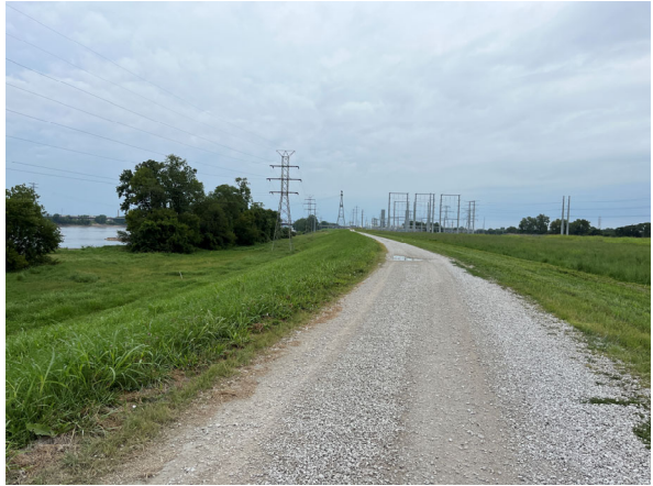
West Embankment, center section
