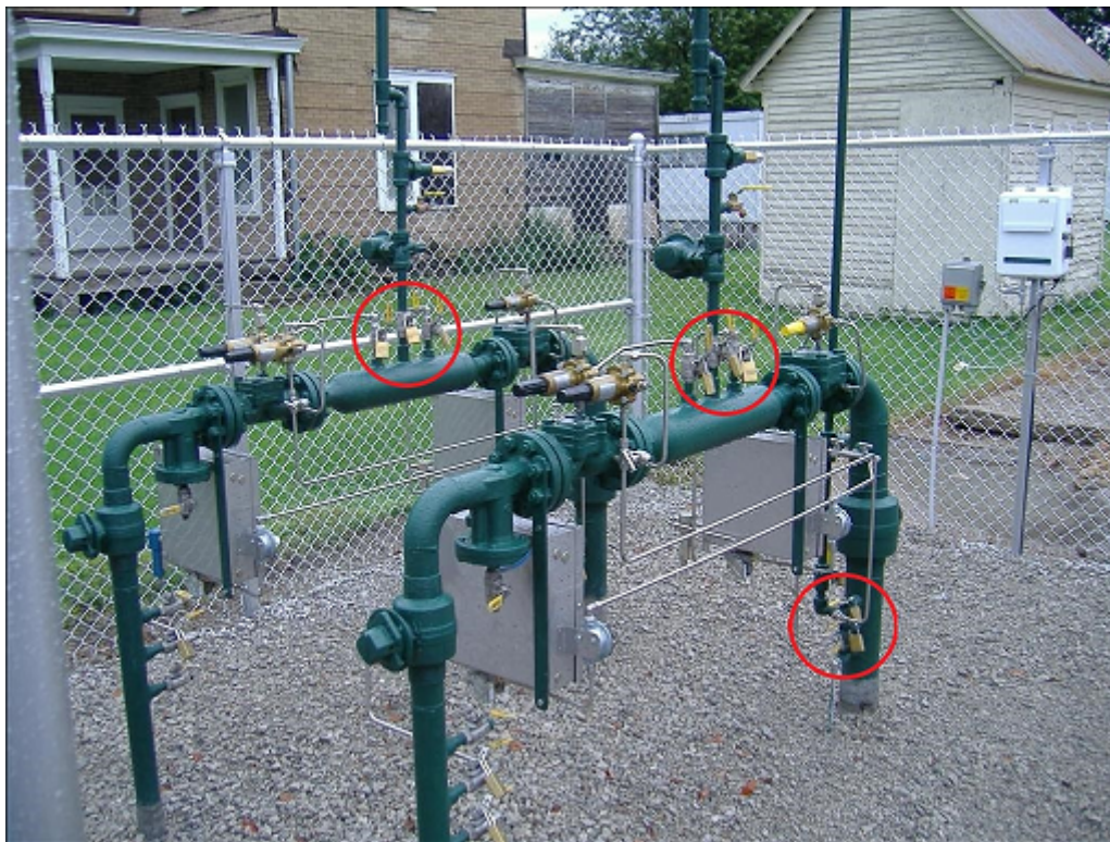
Figure 3: Regulator Station Locking Devices
