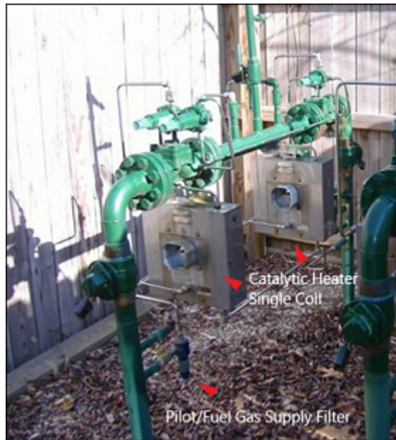
Figure 1: Single Coil Catalytic Heater
