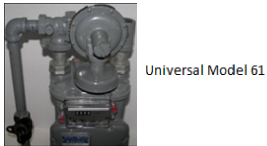
Figure B-3: Regulator with "Regulator Guard"
