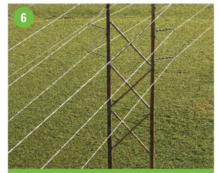
6 Restore easement and energize line
