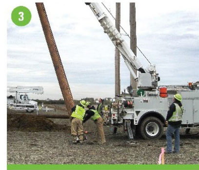
3 Set poles and backfill holes to secure poles in place
