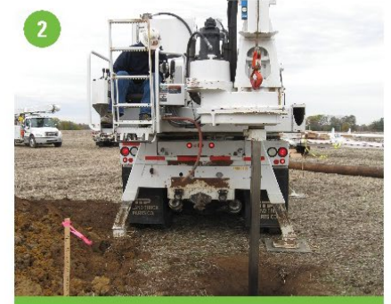
2 Auger holes for new poles
