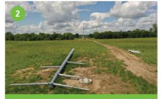
2 Assemble structure on the ground
