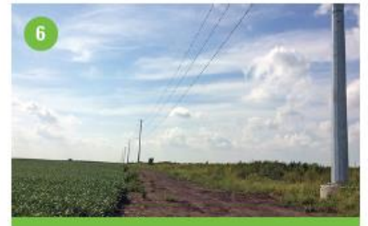
6 Energize line and restore easement
