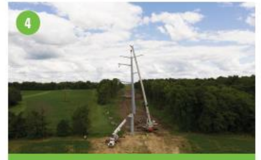
4 Lift structure into hole and backfill with concrete
