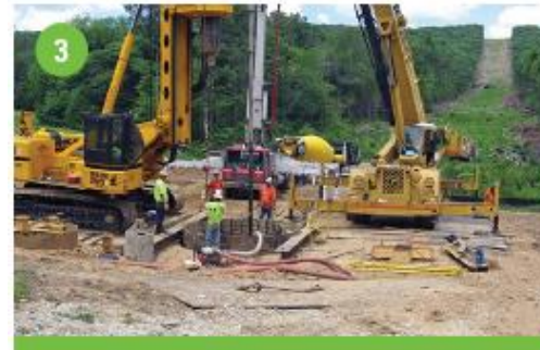
3 Dig structure holes
