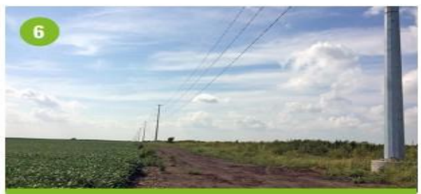
6 Energize line and restore easement
