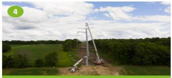
4 Lift structure into hole and backfill with concrete
