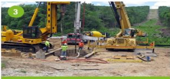
3 Dig structure holes
