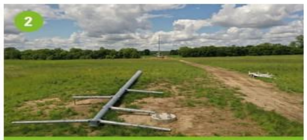
2 Assemble structure on the ground
