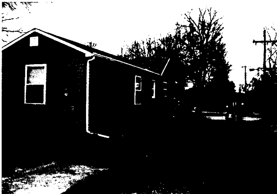
PHOTO 2: View of 304 North 5th Street northeast corner looking southwest from alley. 304-N sampling location to right of building about mid-way along north side. North 5th Street is visible in background.
