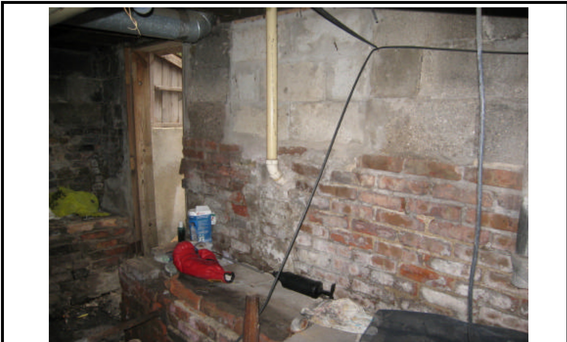
PHOTO 16: View of entrance to basement from south exterior of house.
