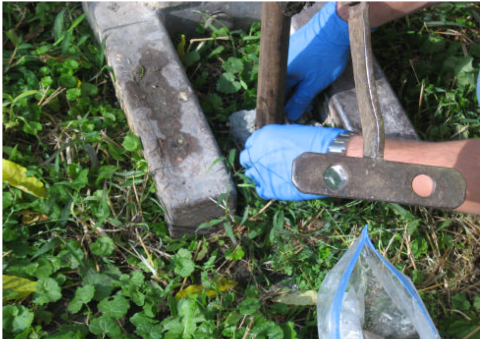
PHOTO 1: View of packing bentonite putty seal around probe.
