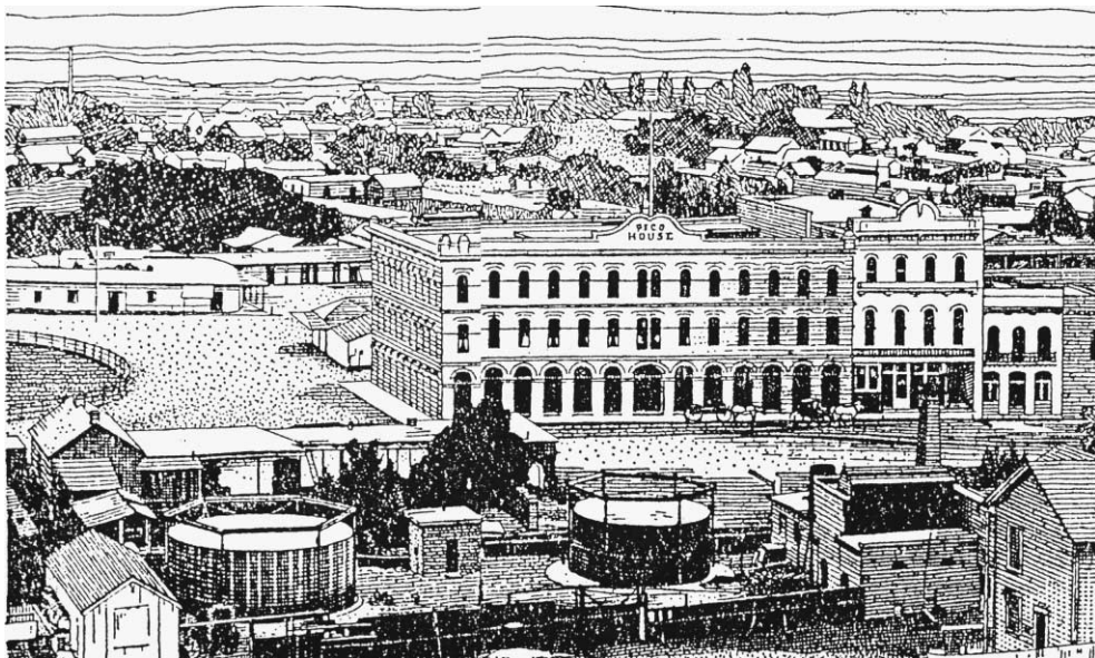
Fig. 1. Los Angeles Gas Company works off Aliso Street at today's historic Olvera Street Plaza. This was a coal-gas plant employing feedstock sent from Australia and from Britain as return cargoes for California grains. The works fronted Governor Pio Pico's hotel and it sported gas lights. Note the two gas holders already present at the 3-year-old plant. In the center is the lime house, storing purification media (from Newcomen Society of America, 1966).
