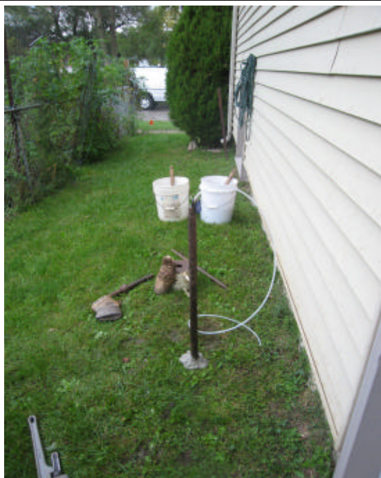
PHOTO 2: View to North along west side of 505 E. Washington at location of VP505EWASH-2. Probe in ground, tubing inside probe.
