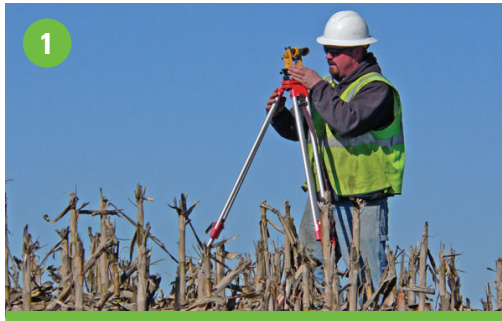
1 Survey structure locations, soil borings and vegetation clearing
