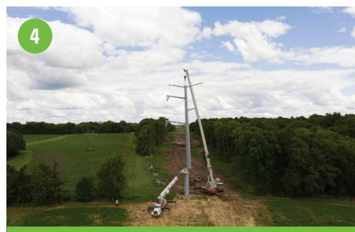
4 Lift and place structure on foundation
