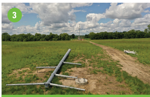
3 Assemble structure on the ground
