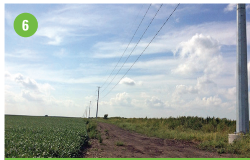
6 Restore easement and energize line
