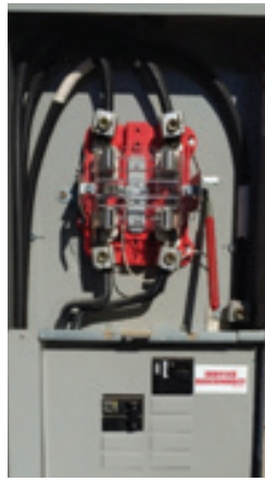
200 Amp With Lever Bypass and Main Disconnect
