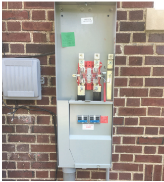
400 Amp With Lever Bypass and Main Disconnect
