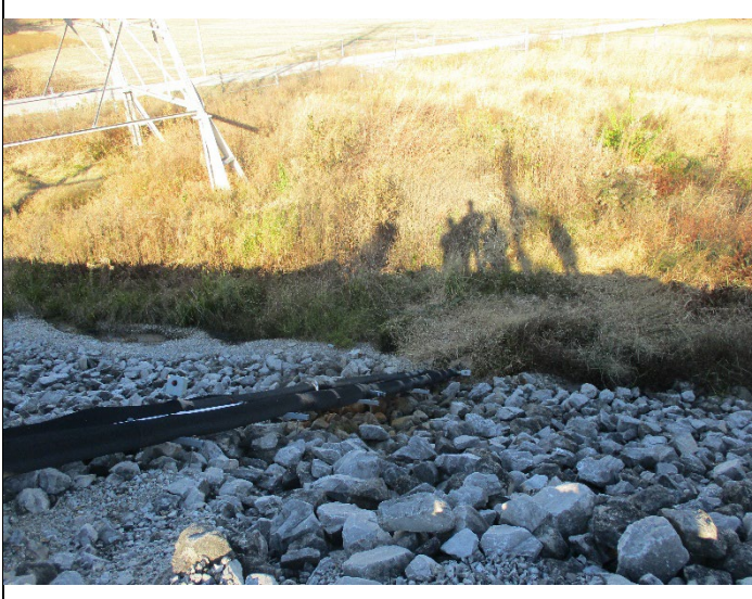
Photo #: 6 Taken by: Maher, Christopher Entity: Huster Substation Permit: MO0137642 Location: Northwestern Portion of Facility Description: View of discharge line from top of levee berm; facing northwest. Date Taken: 11/3/2023 Media: WPC
