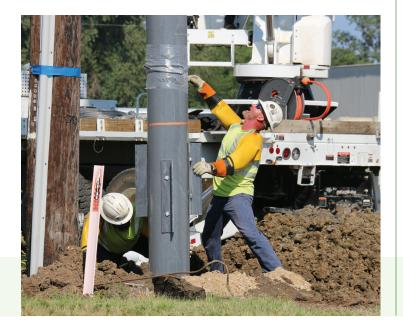
Ameren Missouri maintains more than 4,000 miles of overhead subtransmission lines. Thanks to system hardening upgrades through the Smart Energy Plan, we are addressing some of the oldest and most at-risk circuits in the state — upgrading aging wood poles and adding composite poles to support greater reliability, especially during storms.
