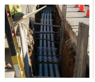
We are upgrading aging underground cable, much of which is at least 40 years old. Due to degradation from direct contact with the soil, we are upgrading the cable and adding protective conduit, which will help to prevent outages and continue to support the reliability of the energy delivery system.
